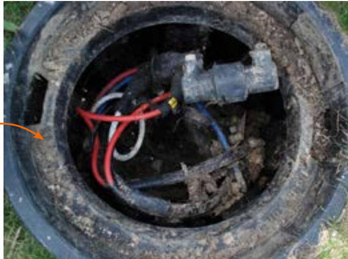
K199 -Installation in a pit
