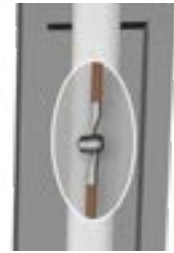
Earth disconnection kit to unbolt
