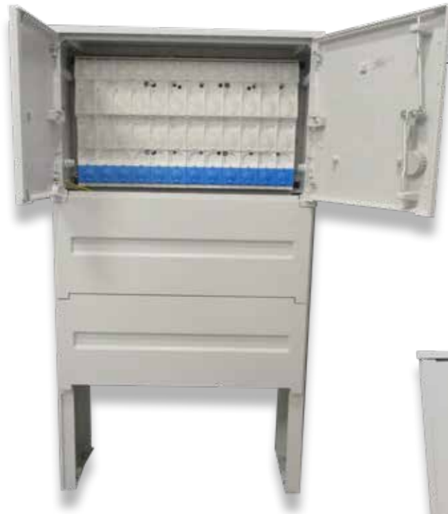
600 cabinet: 12 connection terminals
